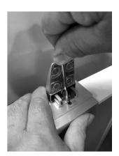
Open the mouth of the assembled bracket and place over the existing wall. Pinch together until firm hold on the wall and tighten the screw. Place roughly 4"-8" from the edge of the existing panel. Repeat process for the second bracket.
